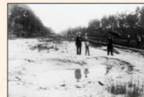
An example of a sand blow, generally referred to as liquefaction, associated with the Charleston 1886 Earthquake.
